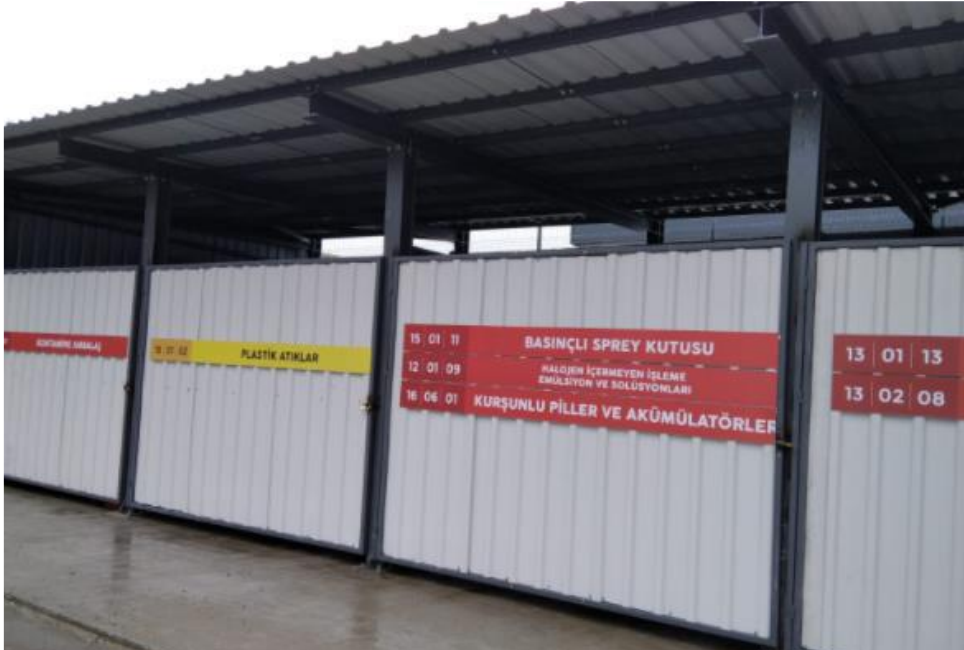
Picture 7: Temporary Waste Landfill
