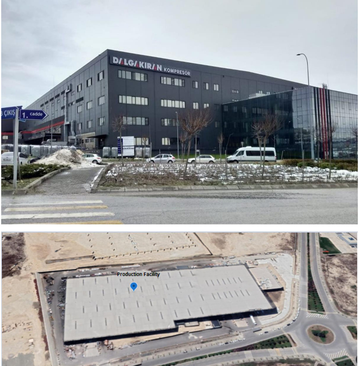
Picture 1: Dilovası Production Facility
